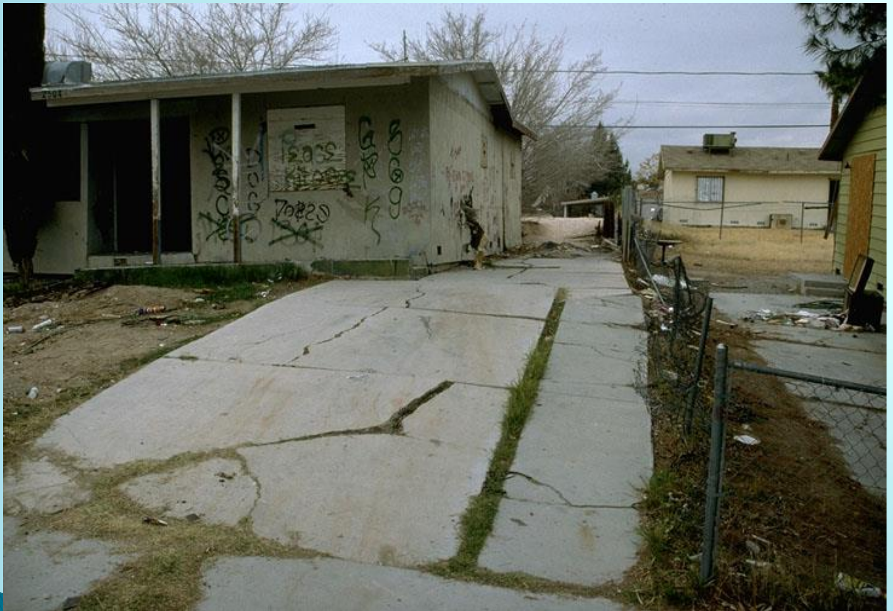
Soil subsidence due to groundwater pumping
